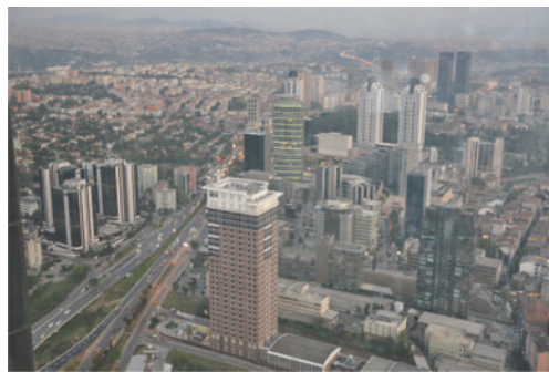
Figure 3. Levent high-rise blocks and the Levent's former social housing units on the left, and illegal housing areas on the right.
