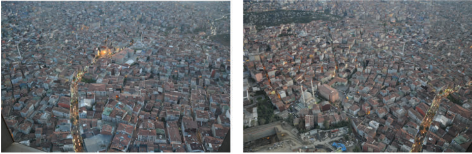
Figure 5. Informal settlement areas: Celiktepe neighbourhood on west side of the Levent-Maslak axis.
